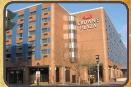
View from building entrance across Falls St.
